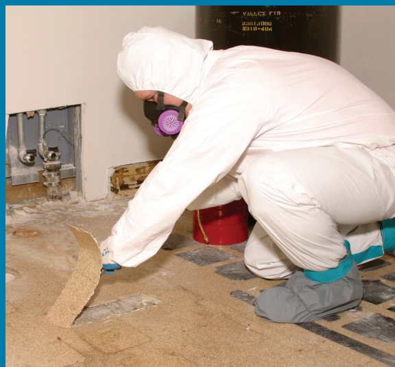
Asbestos Flooring removal
